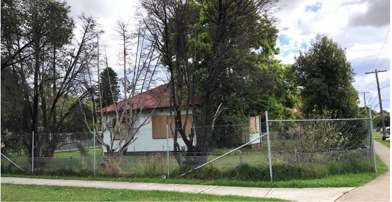
Figure 7: 1 Anderson Avenue, Liverpool Source: CPS, October 2019
